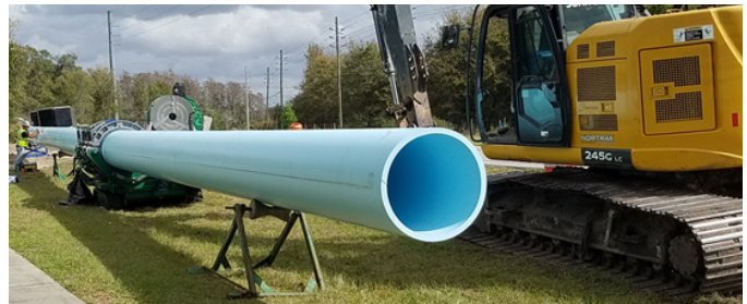
Pipes supported on rollers during fusion operations
