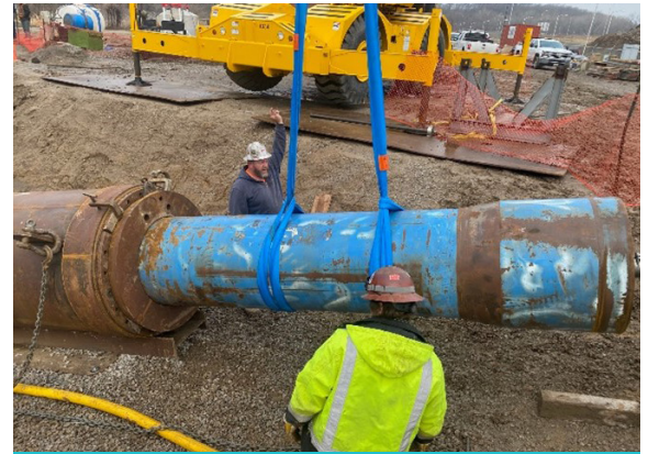
Pneumatic hammer attached to steel casing pipe for installation
